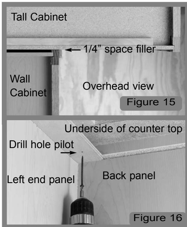
A filler trimmed to 1/4" in thickness or scribe moulding is recommended to conceal the small gaps between the top of the cabinets and the soffit or ceiling.
